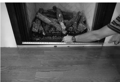
Measure center of firebox
