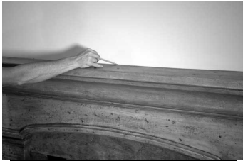
Dry fit shelf and mark the top of the shelf
