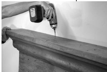
Attach shelf with screws through pre drilled holes
