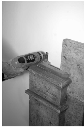
Install L bracket to top of leg and screw to wall
