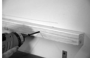
Screw mounting strip to the wall into the studs
