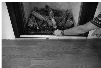
Measure center of firebox
