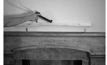
Apply adhesive to the top of the mounting strip
