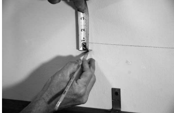
Place another mark below the top mark the thickness of the top
